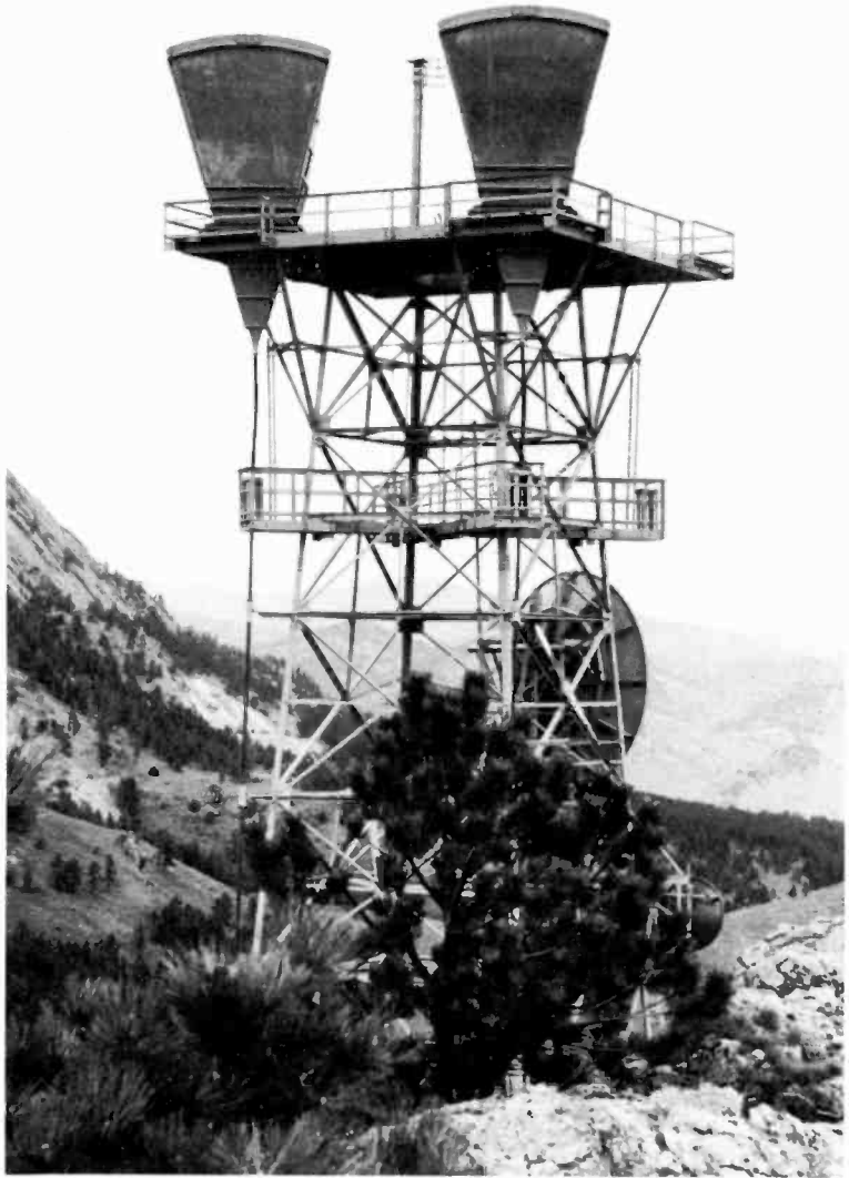
New “horn” type of reflectors on top of the tower; “dish” reflector at the lower level.
